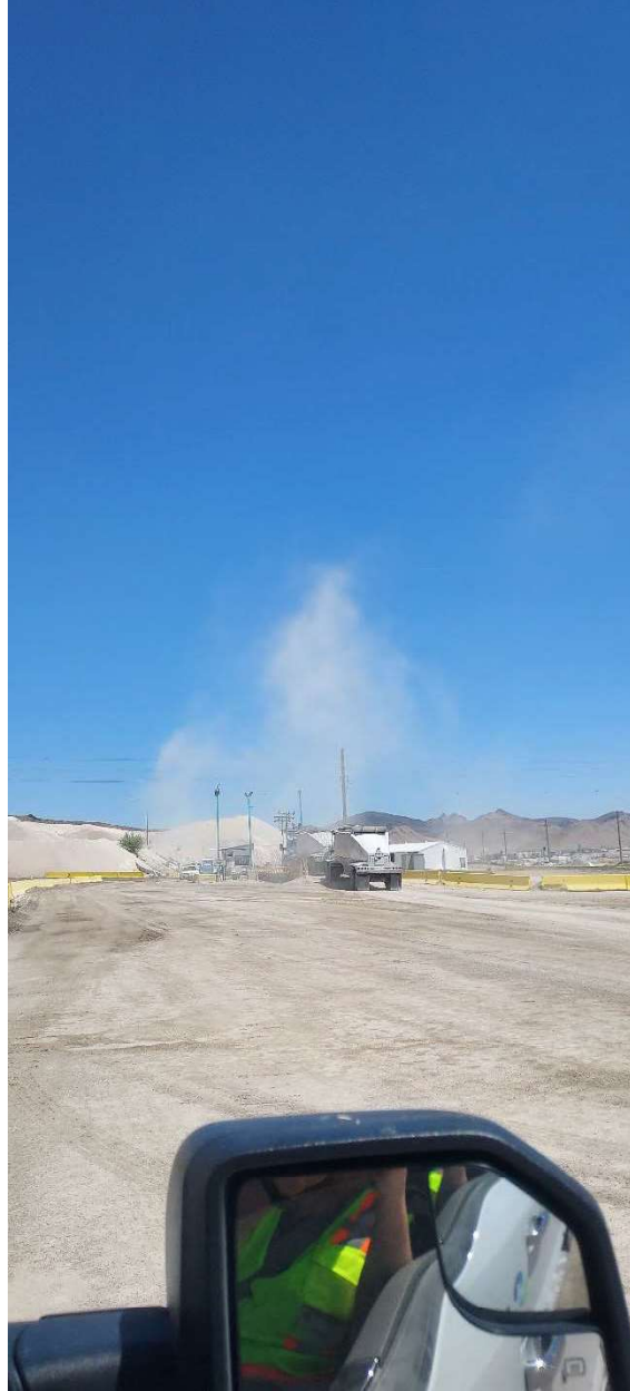
Photograph 1: View of fugitive dust created by haul truck on Haul Road (EU: H06). [Photo taken by Joshua Frye]
